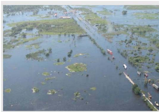
Fig.1: Federal road 180D totally submerged. Transit problems complicated evacuation and emergency aid activities. Source: CENAPRED
